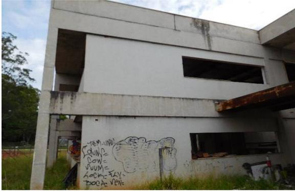
A photograph of a concrete building facade. The building has a modern, industrial look with large rectangular openings. There is a visible horizontal joint in the concrete, and a small displacement is noted. Some graffiti is visible on the lower part of the wall. | Fachada lateral esquerda<br>Parte frontal<br>Vista geral<br><br>1-Deslocamento de junta de movimentação horizontal |
