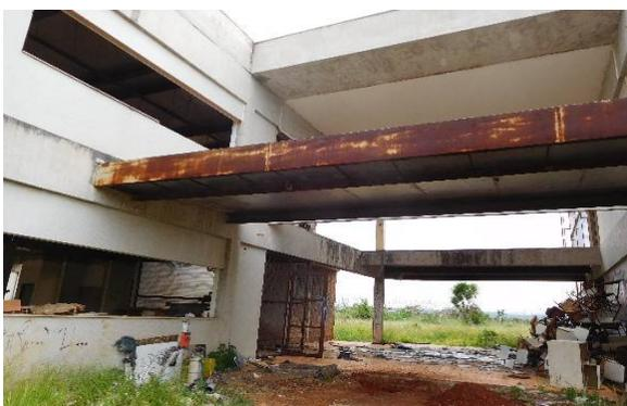
A close-up photograph of the rusted metal canopy structure, showing the extent of the surface oxidation and the structural details.                                                                                                                                   | Fachada frontal<br>Lado esquerdo<br><br>1-Detalhe da anomalia anteriormente descrita                               |
