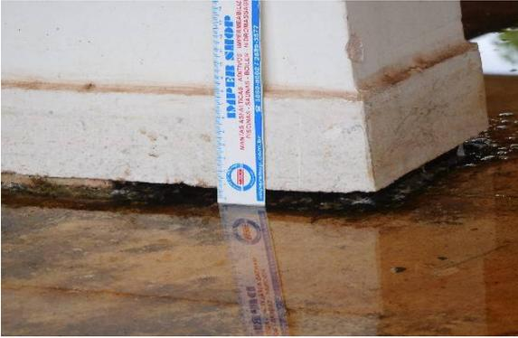
A close-up photograph of a concrete wall base. A blue and white ruler is placed vertically against the wall to measure a horizontal deformation. The ruler shows a measurement of 2.5 cm. The wall is light-colored and shows some staining and wear at the base.                                                    | Segundo pavimento<br>Ponto 23<br><br>1-Medição da deformação. e = 2,5 cm |
