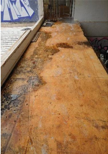
A photograph showing a concrete floor surface with several dark, transverse cracks. The floor appears aged and somewhat stained. In the background, there is a blue and white patterned wall or fence.                                                 | Segundo pavimento<br>Ponto 50 - Piso<br>Piso<br><br>1-Fissuras transversais             |
