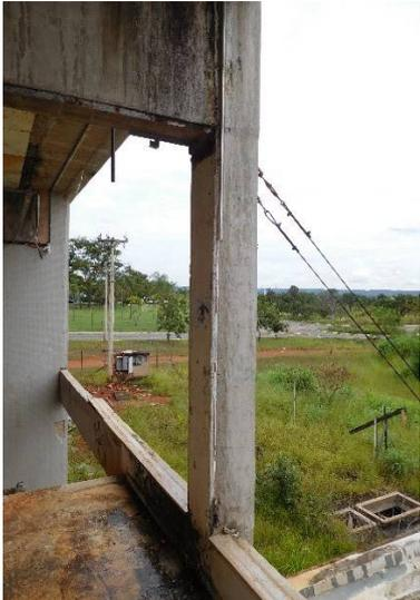
A photograph of a concrete pillar supporting a structure. The base of the pillar shows signs of damage, including chipped concrete and exposed aggregate. The pillar is situated outdoors, with a grassy area and a fence visible in the background. | Segundo pavimento<br>Ponto 52 - Pilar<br><br>1-Concreto danificado pontualmente na base |
