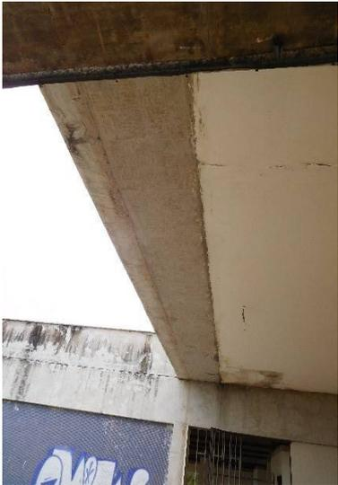
A photograph taken from below, looking up at a concrete ceiling. A prominent vertical crack is visible in the concrete slab. The surrounding area shows some discoloration and wear.                                                                  | Segundo pavimento<br>Ponto 51 - Teto<br>Vista                                           |
