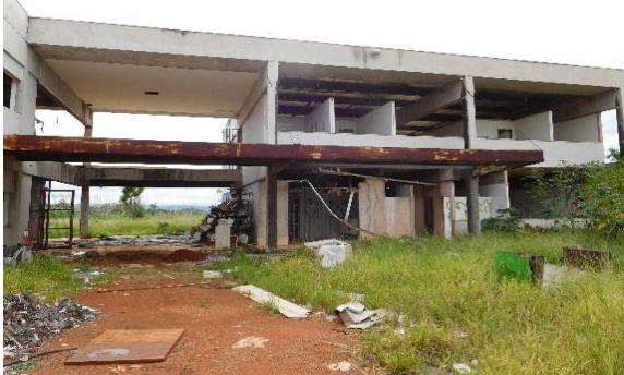
A photograph showing the front of the building from a low angle, highlighting a metal marquee with significant rust.                                 | Fachada frontal<br>Lado esquerdo<br>Vista geral<br><br>1-Marquise metálica com oxidação superficial generalizada    |
