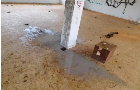
A photograph showing a concrete floor slab with significant deformation and cracking. A white support column is visible on the left, and a small metal box lies on the floor near the center.   | Segundo pavimento<br>Ponto 26 - Piso<br><br>1-Deformação da laje de piso<br><br>2-Fissuras em diversas direções                               |
