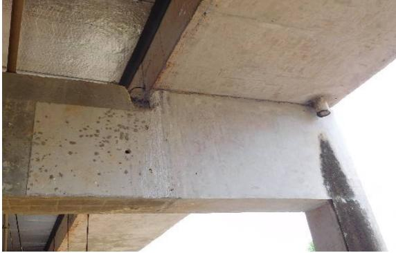
A photograph showing a concrete wall and ceiling. The concrete appears damaged, particularly near the bottom, likely for the installation of a Surface Protection and Drainage System (SPDA). | Segundo pavimento<br>Ponto 29<br><br>1-Concreto danificado para instalação de SPDA                                                            |
