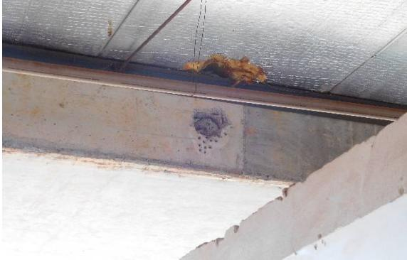
A photograph showing a close-up of a concrete wall and ceiling. The ceiling has a hole with debris, and the wall shows signs of damage and discoloration.                                     | Segundo pavimento<br>Ponto 28<br><br>1-Concreto danificado pontualmente<br><br>2-Revestimento termo acústico da telha danificado pontualmente |
